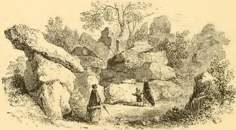
Part of the Rock-work—the Rocky Postal.
